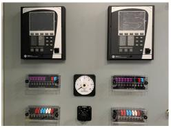
The interior of the custom enclosure is integrated using wireway or conduit per the customer requirements. The custom enclosures can be designed to include low-voltage or medium-voltage electrical equipment, protective relay panels or designed as a sound attenuated generator enclosure. Site conditions are considered in the structural design criteria, as well as HVAC heating and cooling requirements.
