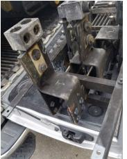
The existing bus had a failure when it shorted the bus phase-to-phase. This customer needed the bus duct rebuilt to match the existing, obsolete bus duct. It was the final length of bus duct that connected to the distribution switchgear, and there was no time to manufacture a complete run of bus duct.
